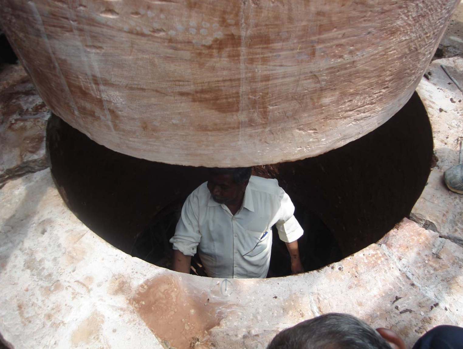
Fixing of Key stone for 1st dome, September 2006 – Completion of Masonry dome with clear span of 85.15 meter, largest ever in masonry
