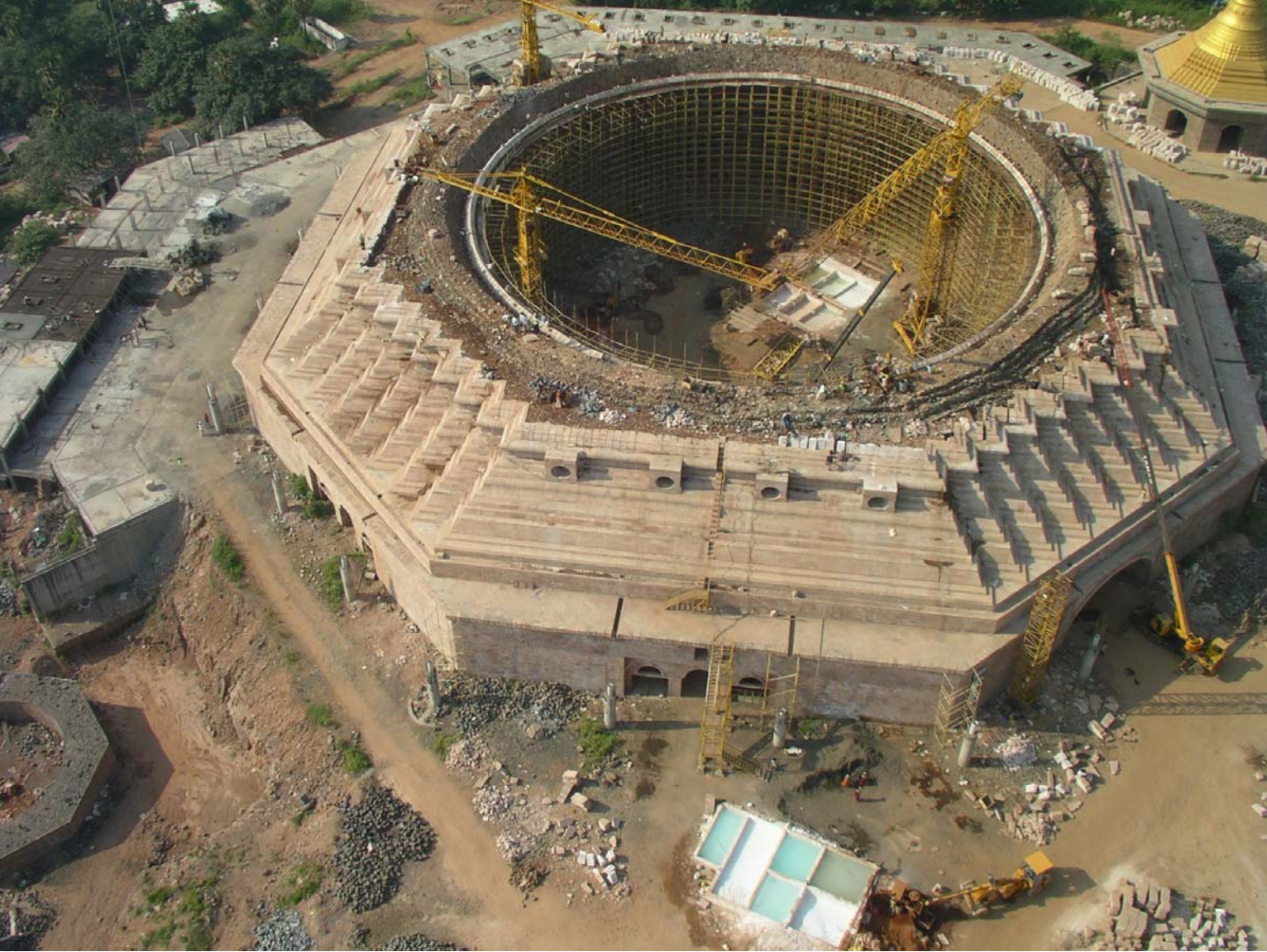
Placing of crane over structure itself
