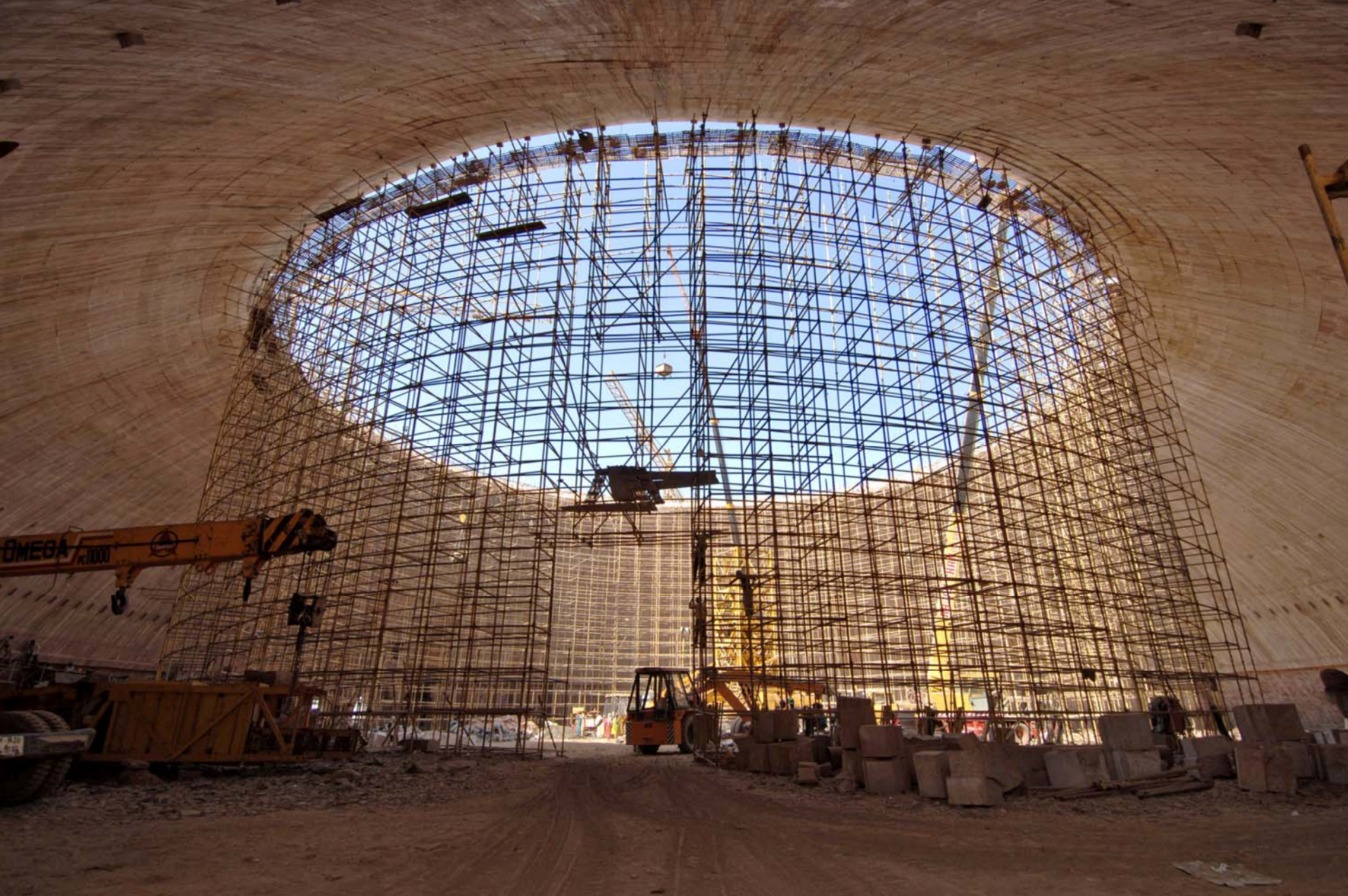
Work in progress without centering
